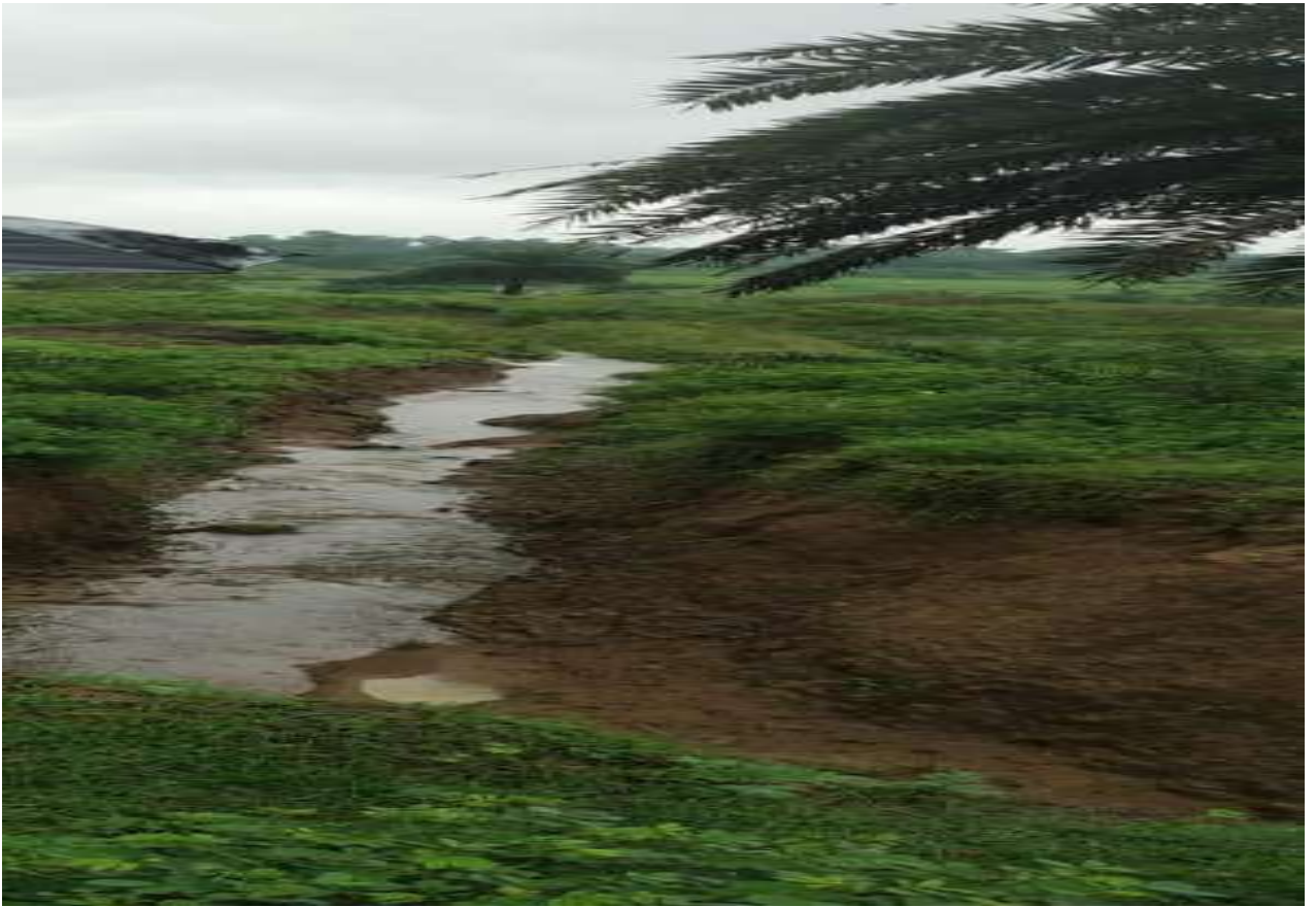
GARLAND DRAIN AT PARBALI AND DUBESWARI
