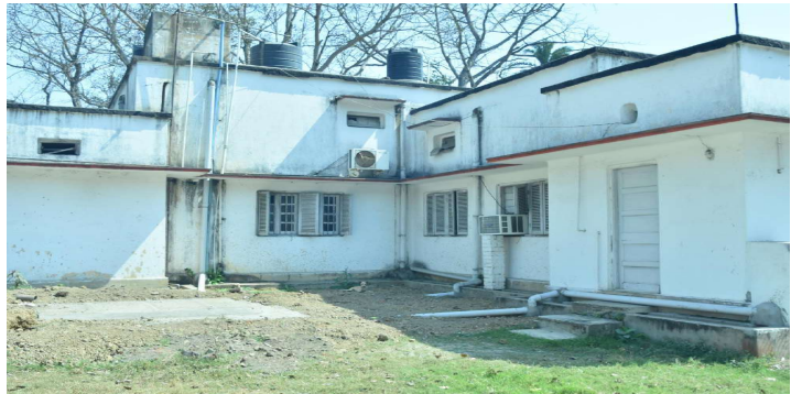
Rain Water Harvesting at Chinakuri Guest House
