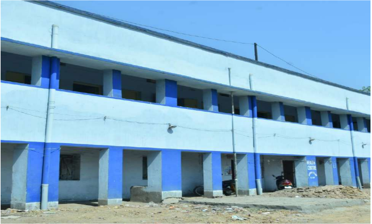
RAIN WATER HARVESTING AT PARBELIA AGENT OFFICE BUILDING
