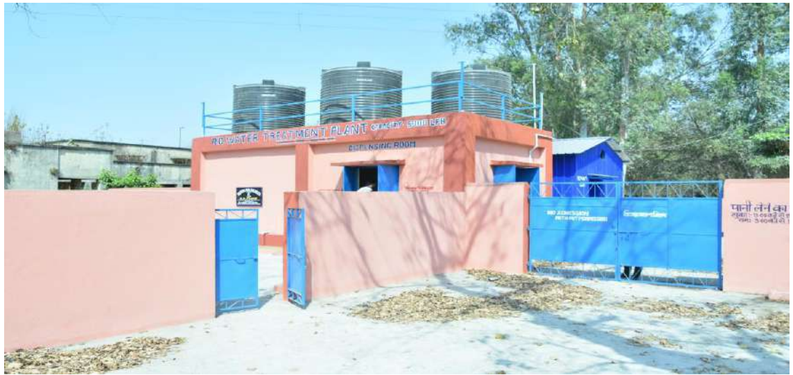
RO PLANT AT CHINAKURI MINE I
