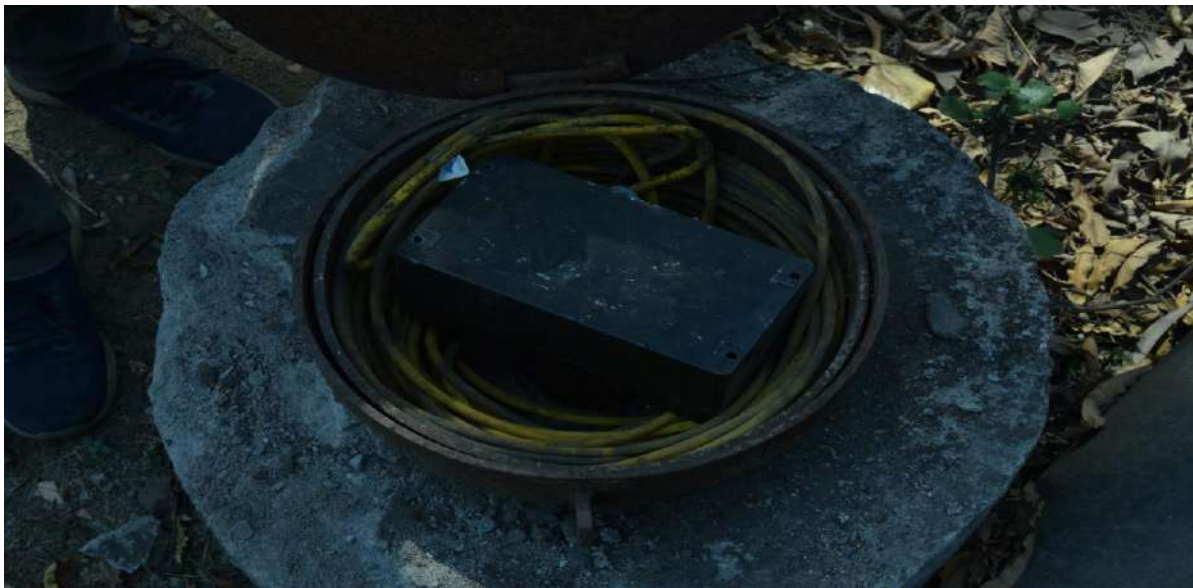
Piezometric Borewell with Automatic Well Recorder at Sodepur 9/10 Pit.
